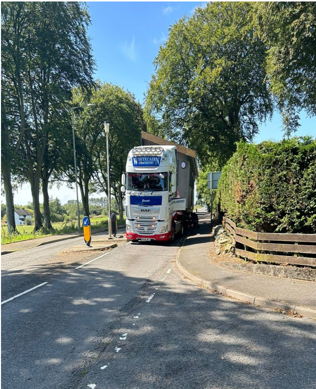
The new Dunragit community hub cabin arriving on site in Orchard Road.
